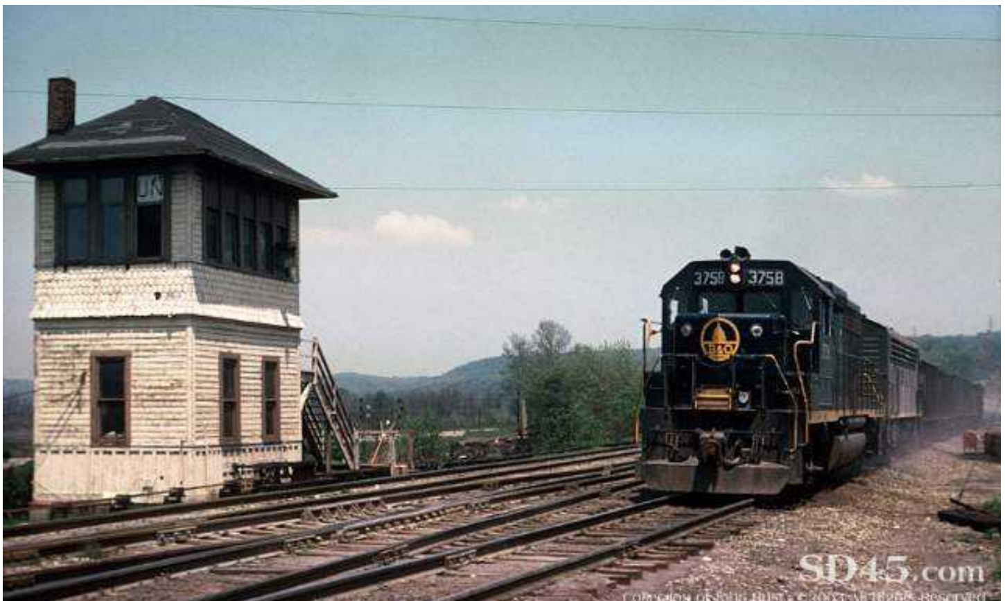
UN Tower and B&O 3758 in May 1975.
